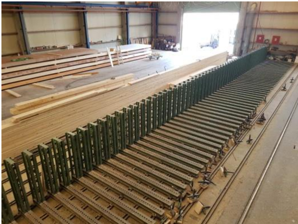
Figure 5b: Another view of the press of a length of 30 m.
